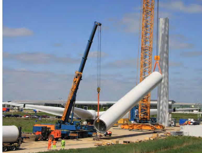
Figure 32: Example of a “tailing operation” with a main crane and a tailing crane
