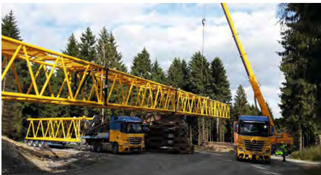
Figure 15: An elevated boom support on a sharply sloping terrain
