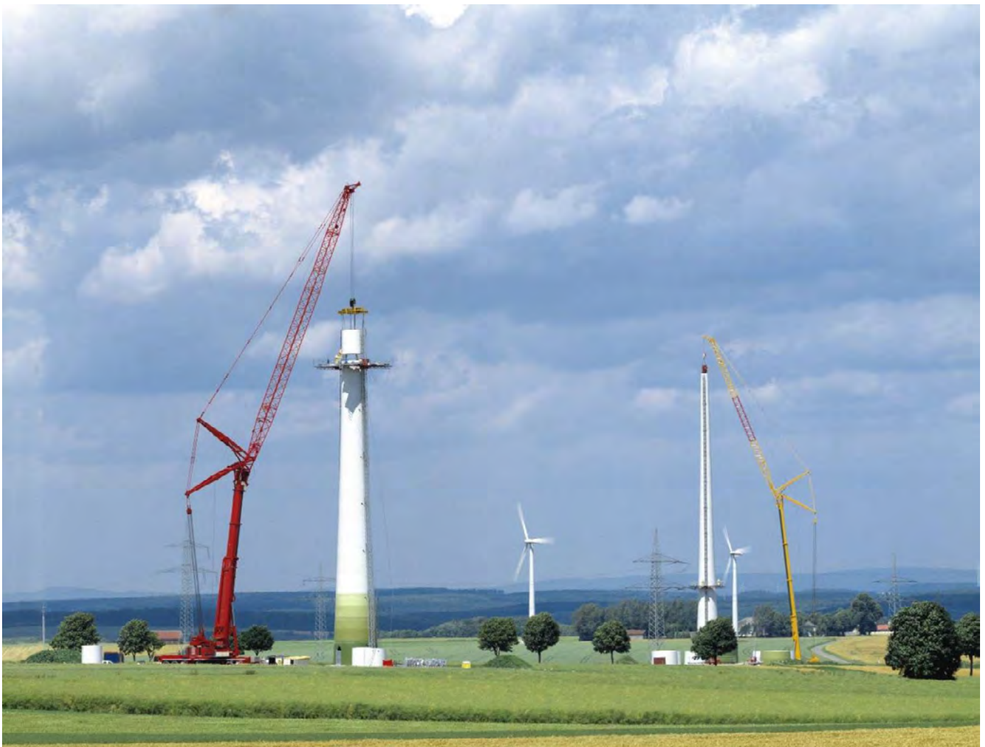
Figure 5: Two 500 tons hydraulic cranes equipped with luffing jib
