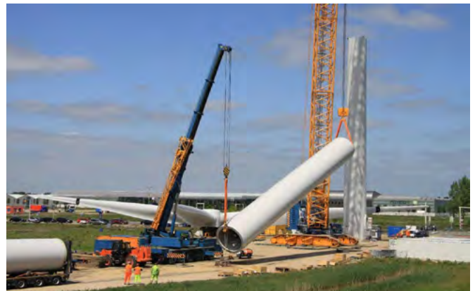
Figure 4: A tailing operation of a tower section
