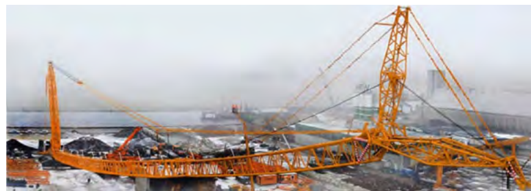
Figure 16: Raising the mast of a 650 ton crawler crane.
