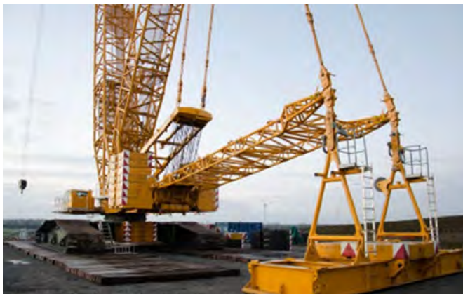
Figure 7: The superlift tray of a 600 tonnes crawler crane.
