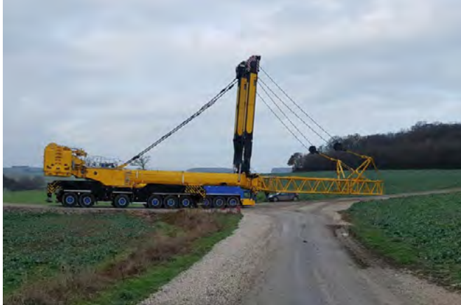
Figure 31: Site transport of a 750 tons Telescopic crane
