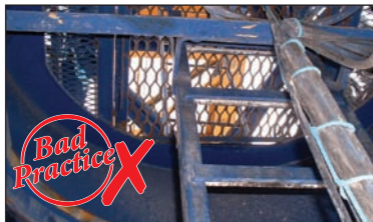
RESTRICTION OF LADDER WIDTH BY CABLES
