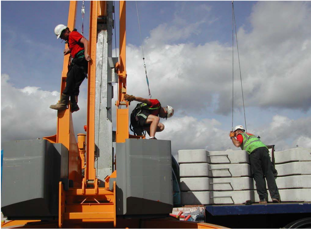
Installing Ballast using Full Harnesses with Inertia Reel Lanyards
