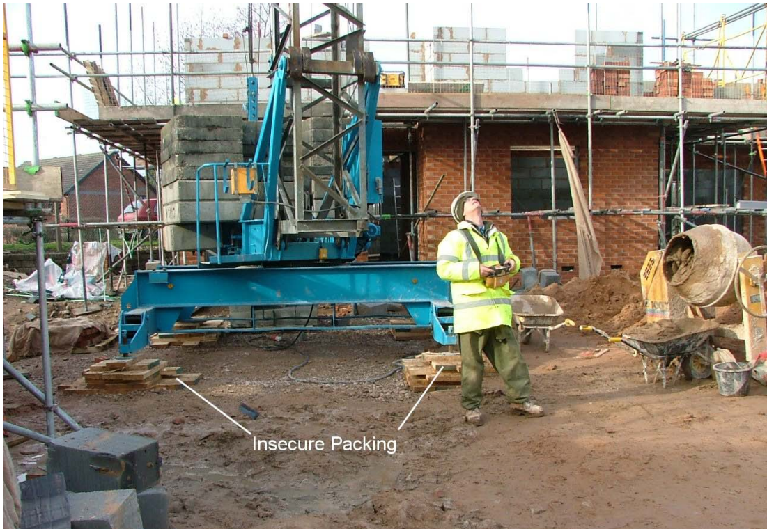
Insecure Packing Under Outriggers (See 5.3)
