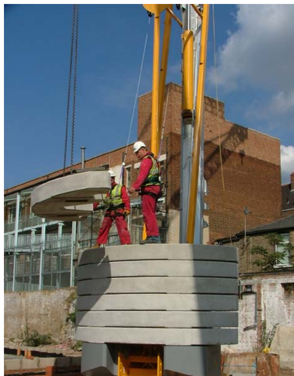
Installing Ballast using Full Harnesses with Inertia Reel Lanyards
