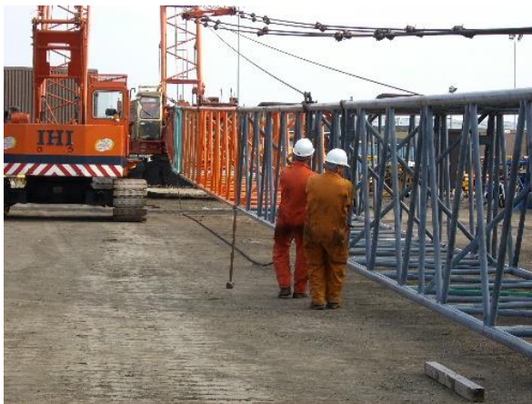
Fig. 3. Extending Rope at Ground Level
