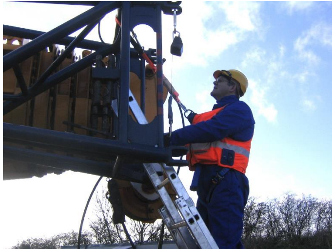
Figure 2 - Work Positioning System
