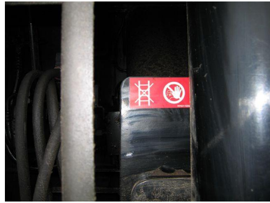
Fig. 2. Additional Access Ladders
