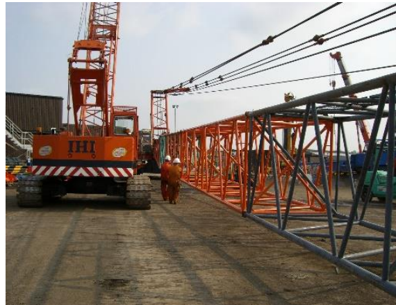
Fig. 2. Extending Rope at Ground Level
