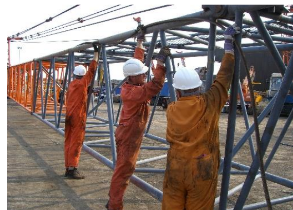
Fig. 6. Lifting Rope onto Jib
