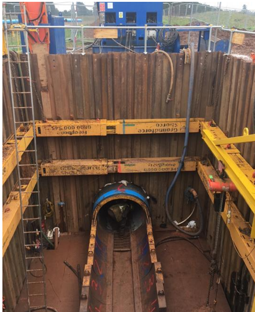
Figure 24 – Braced drive pit for pipe jacking operation
