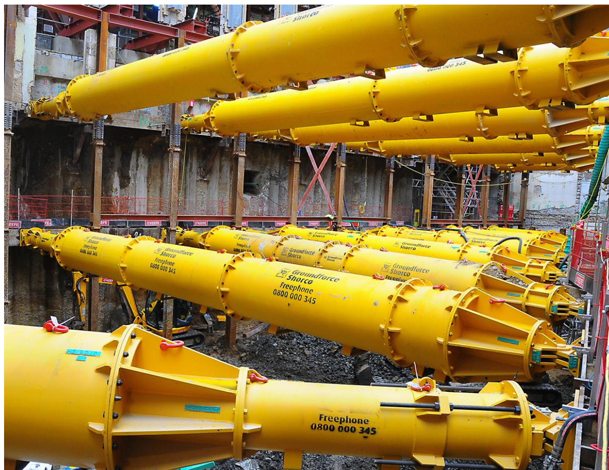
Figure 25 - Struts to concrete piles
