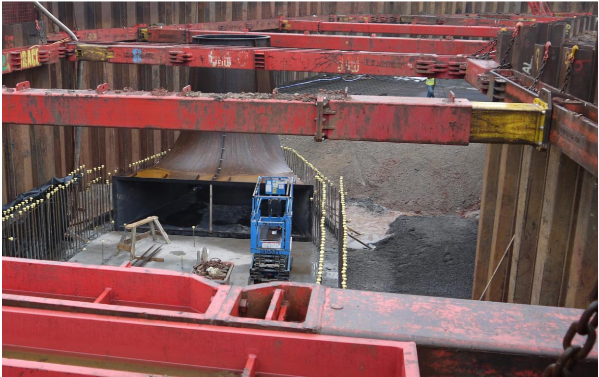
Figure 26 - Struts supporting a bracing frame with sheet piles
