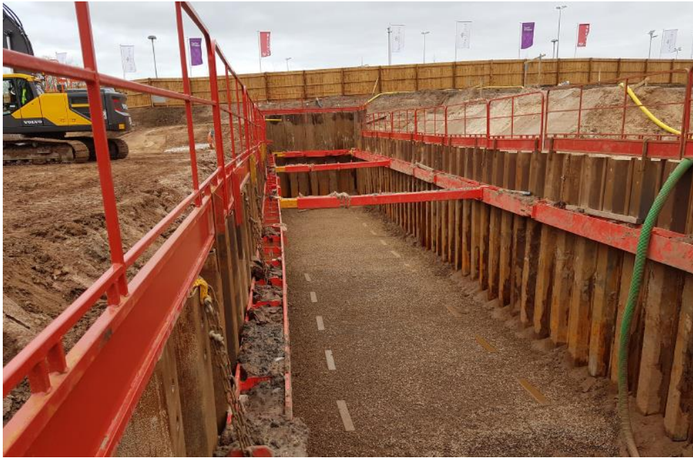
Figure 23 - Cofferdam for storm water attenuation tank on a housing development
