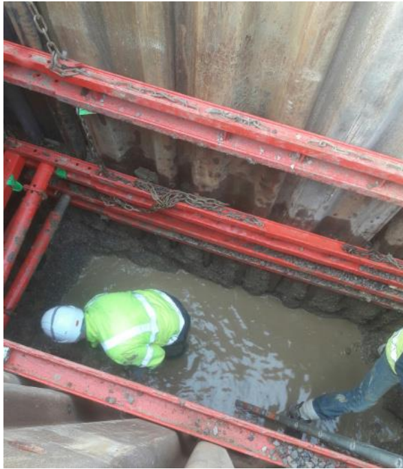
Figure 17 - Sheets and walers for sewer trench
