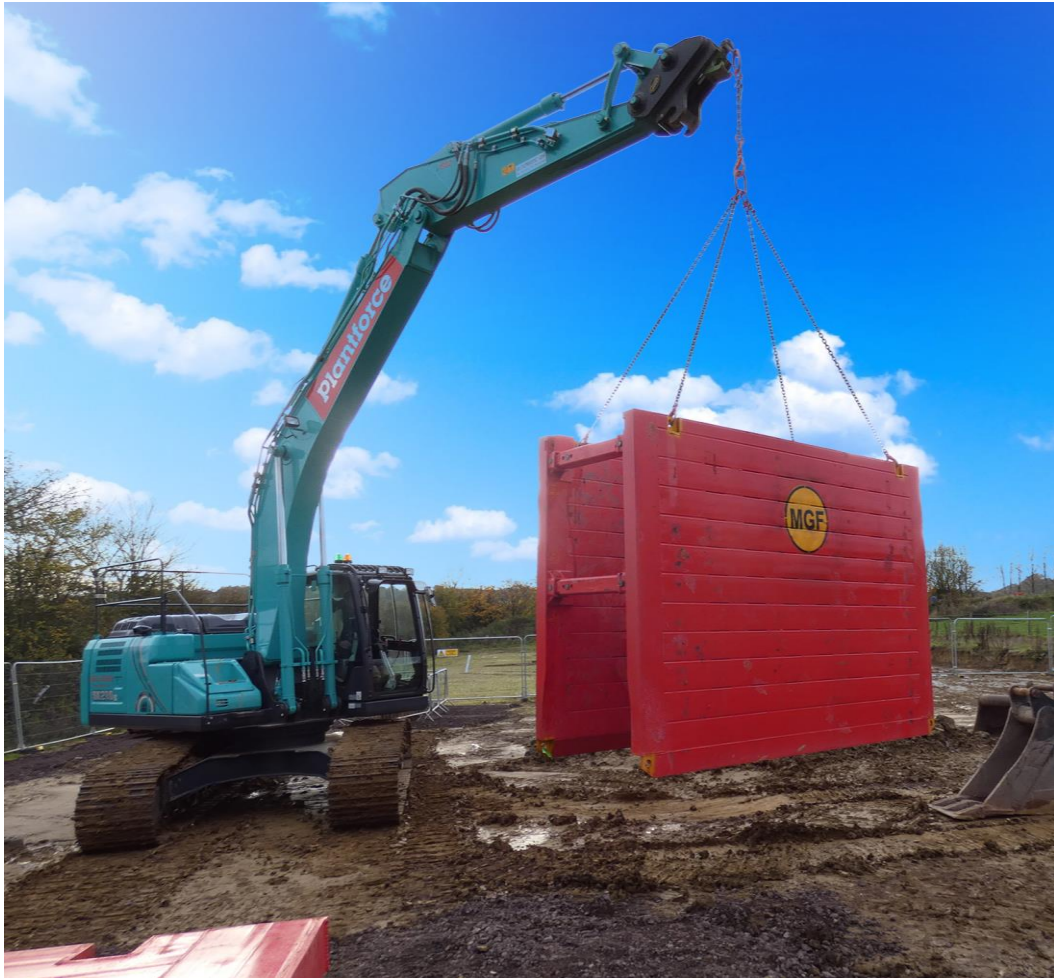
Figure 8 – Trench box during lifting operation
