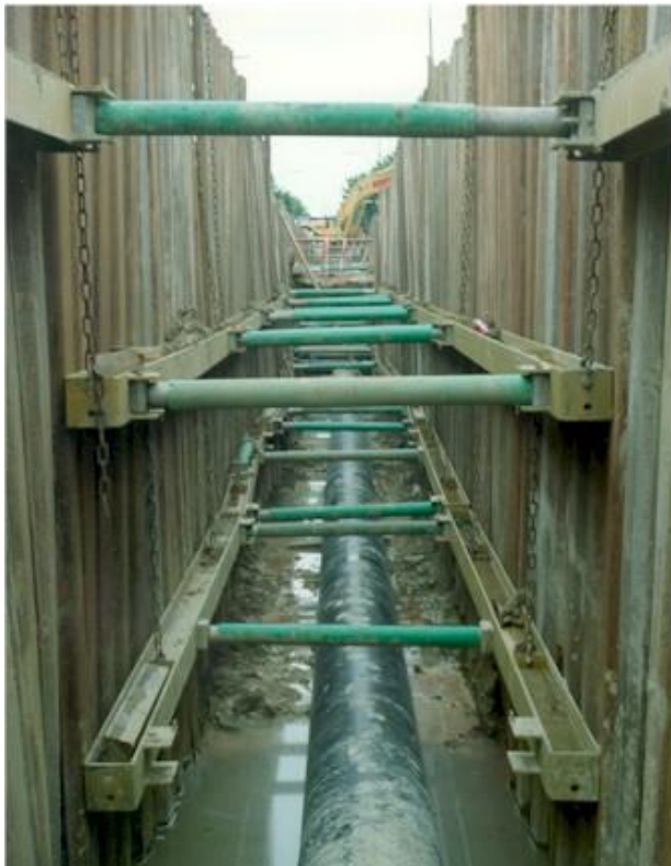
Figure 15 - Trench with Walers
