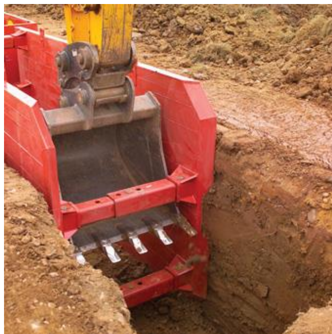
Figure 13 – Drag Box cutting edge
