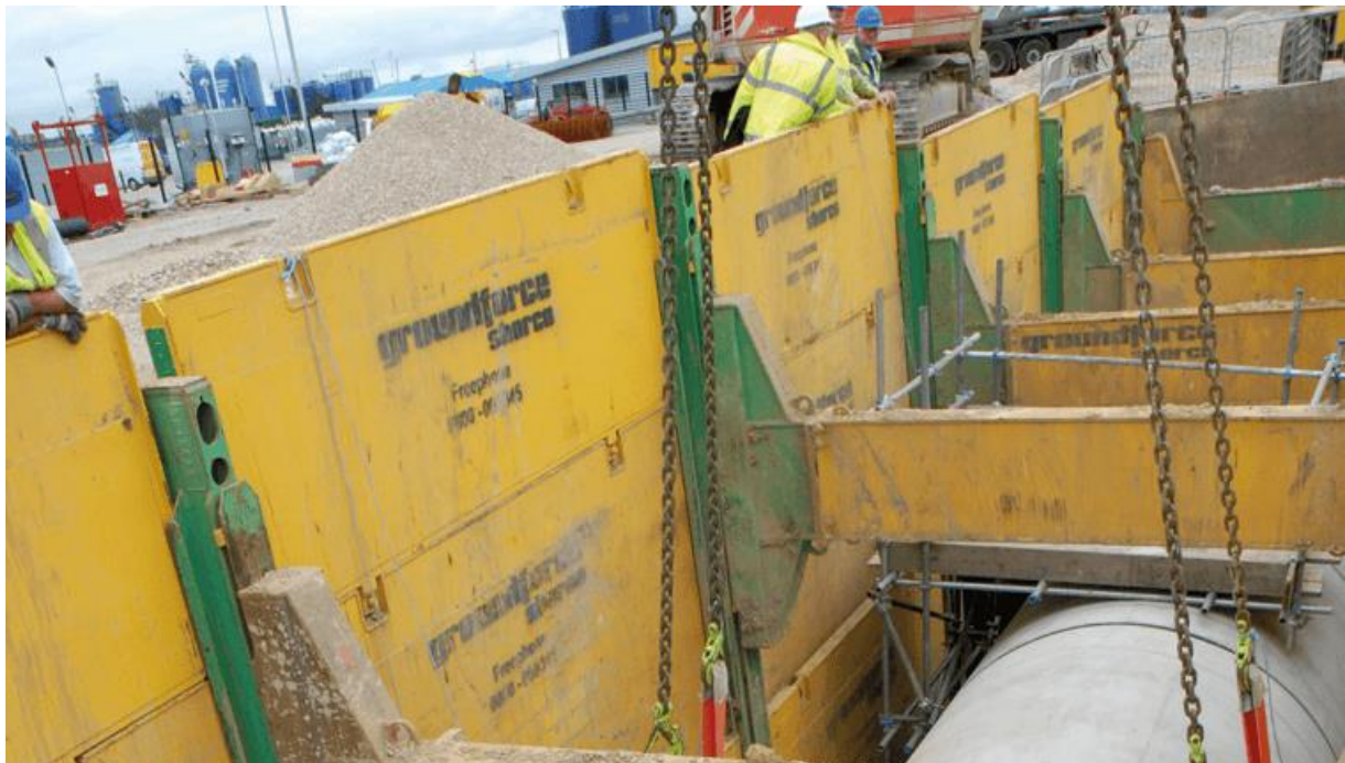
Figure 14 - Slide Rail system
