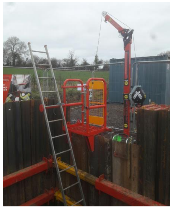
Figure 18 – Manhole brace with access/egress
