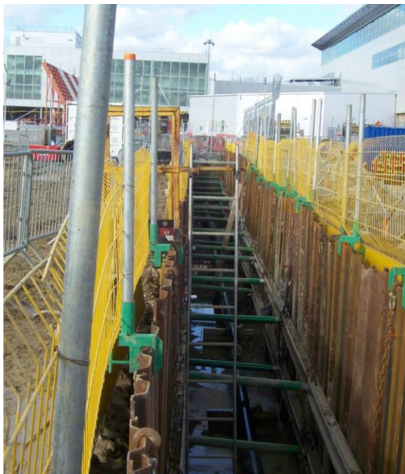
Figure 19 - Sheets and walers for trench run
