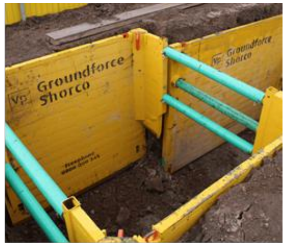
Figure 7 - Typical Manhole Box
