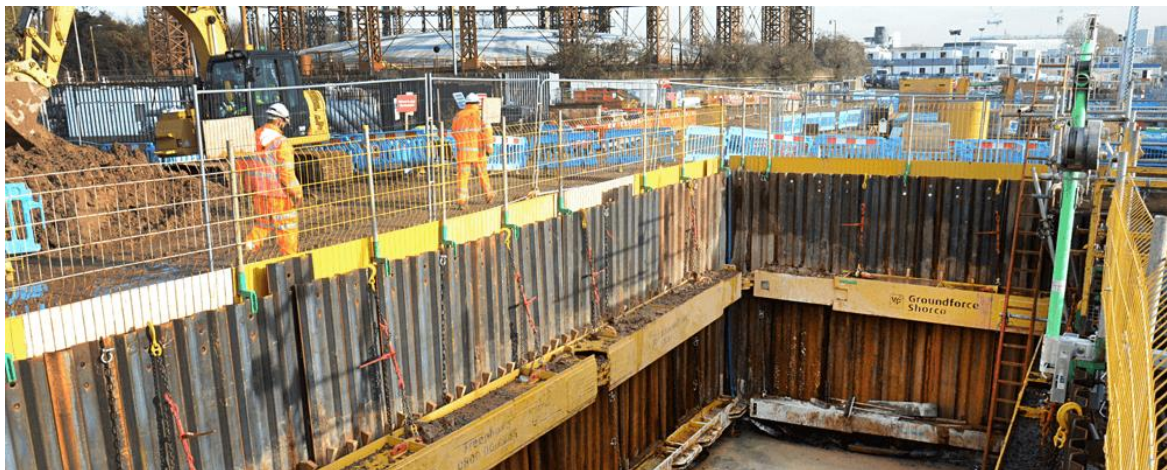
Figure 21 - Large excavation with clear span bracing frames
