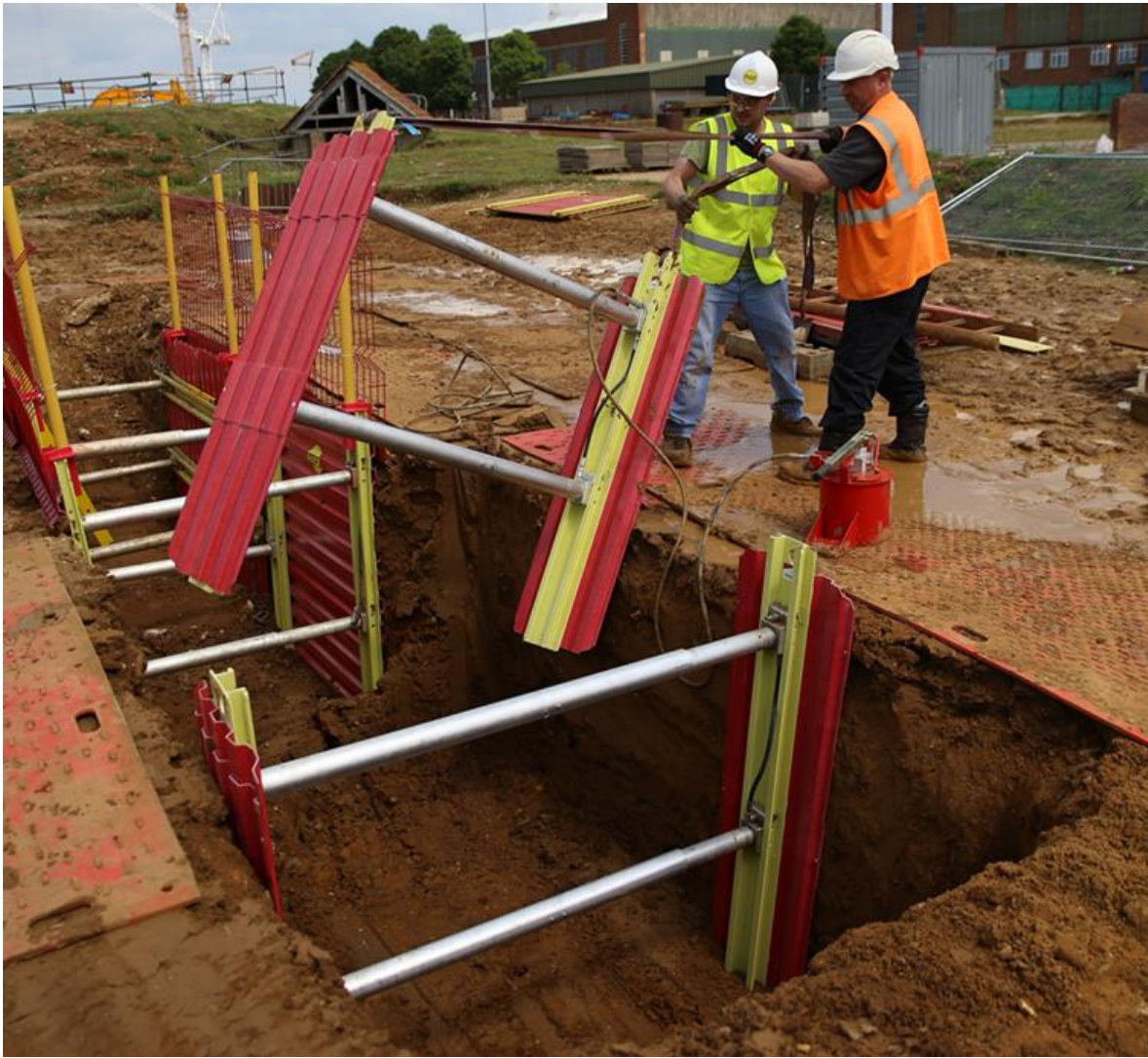
Figure 29 – GRP trench box and Vertishores
