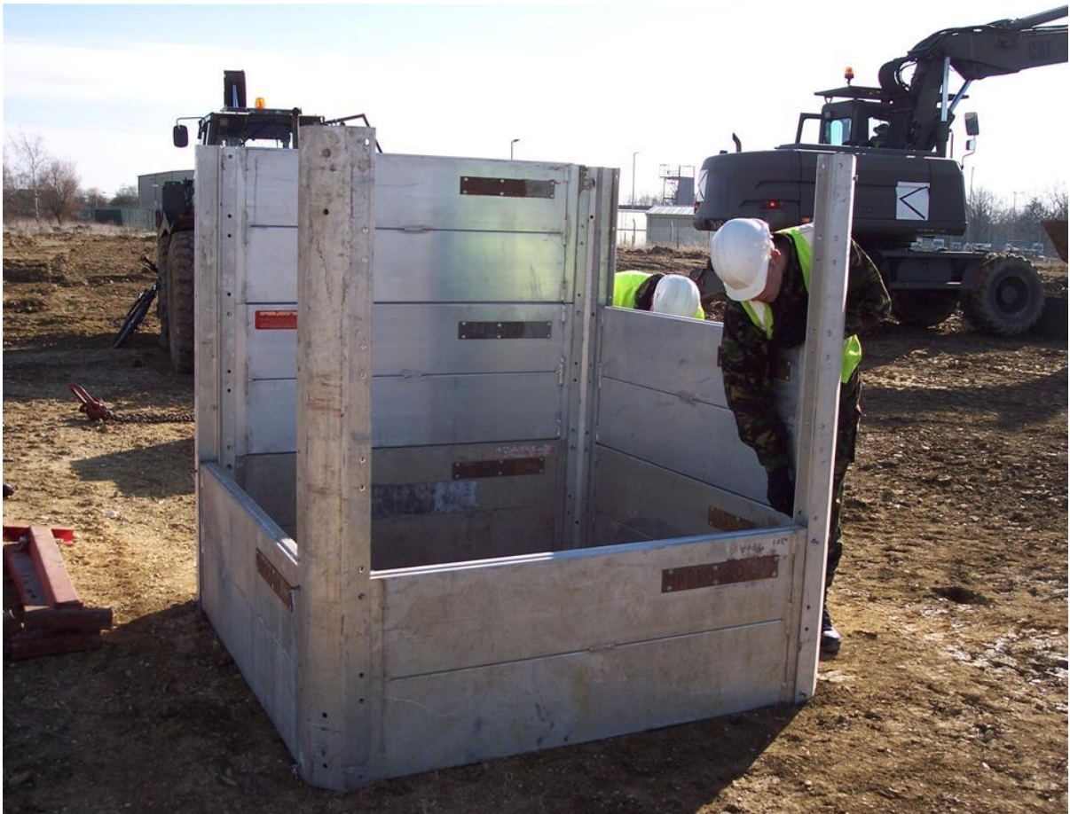
Figure 28 – Modular Aluminium panel system
