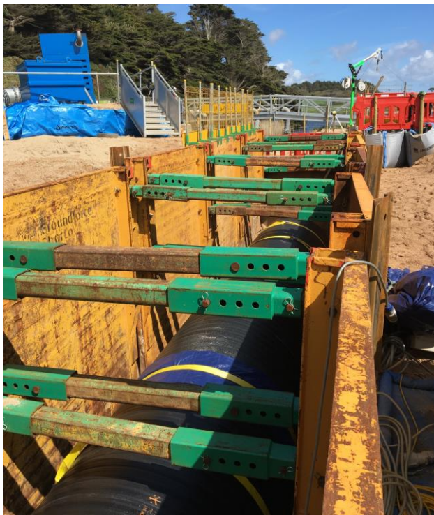
Figure 9 – High clearance trench boxes
