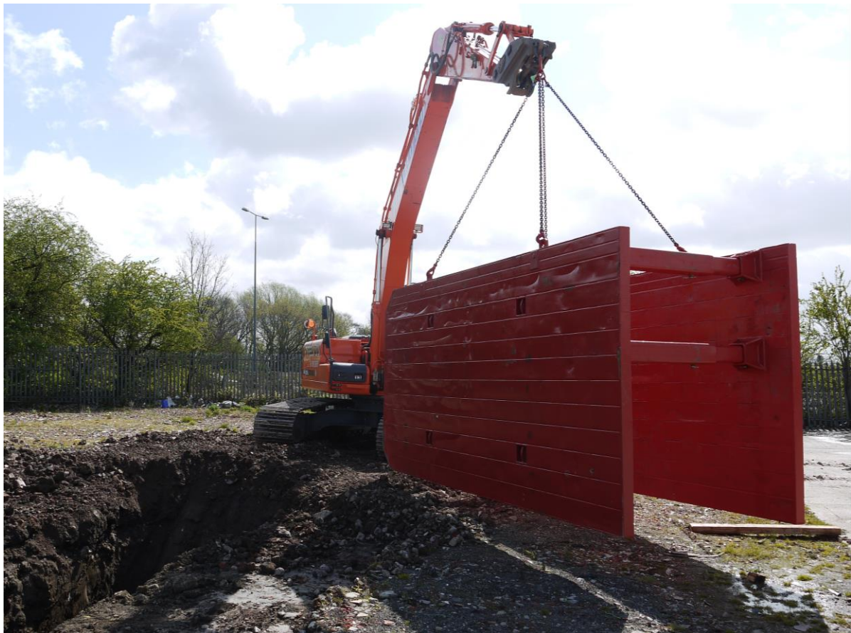
Figure 11 – Lifting Drag Box
