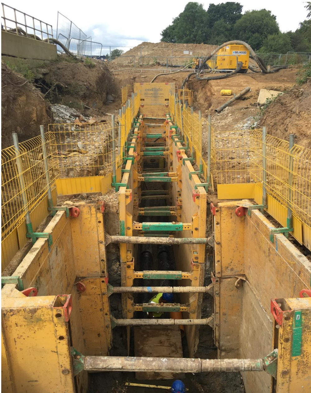
Figure 5 – Trench and Manhole Boxes
