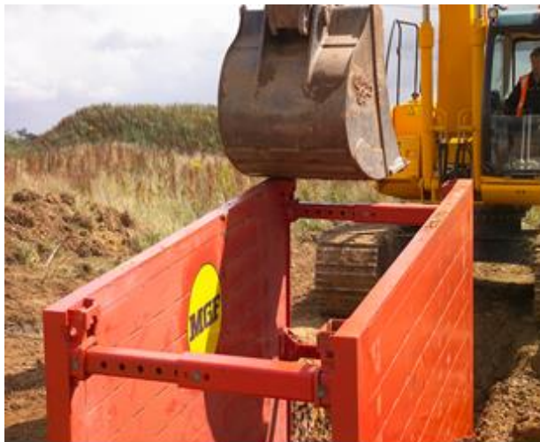
Figure 6 - Trench Box with incremental struts
