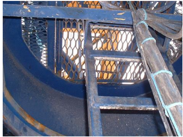
Figure 2 - Cables Attached to Ladder
