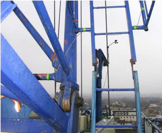
Figure 1 - Uneven Rung Pitch
