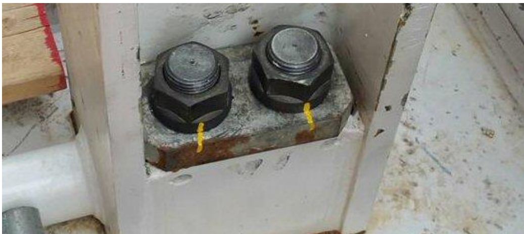
Figure 2 – Marking on Initial Installation
