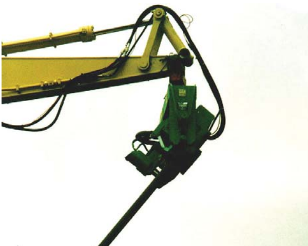
Figure 3.34 ICE SH pitching sheets
