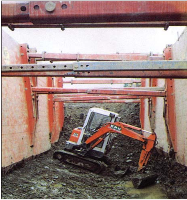
Figure 2.31 Heavy Duty Trench box
