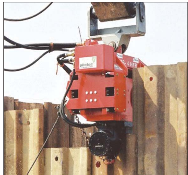
Figure 1.7 Driving trench sheeting with an excavator mounted vibratory hammer
