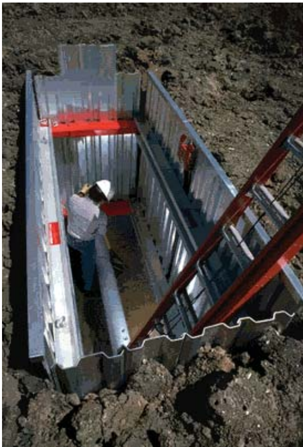
Figure 2.15 Hydraulic Shoring Shield
