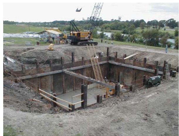
Figure 2.39 King post system (In US)
