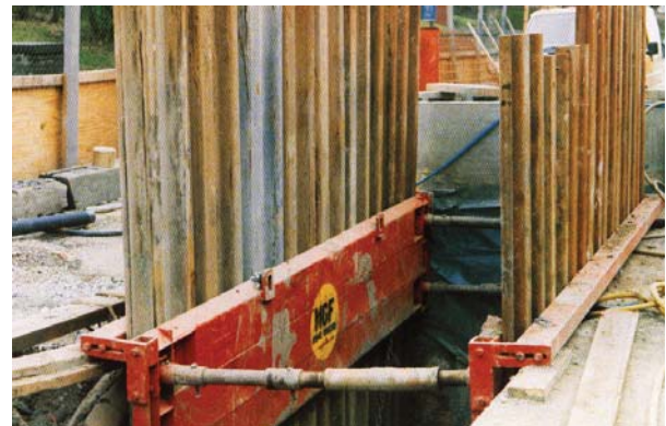
Figure 2.09 Piling Frame
