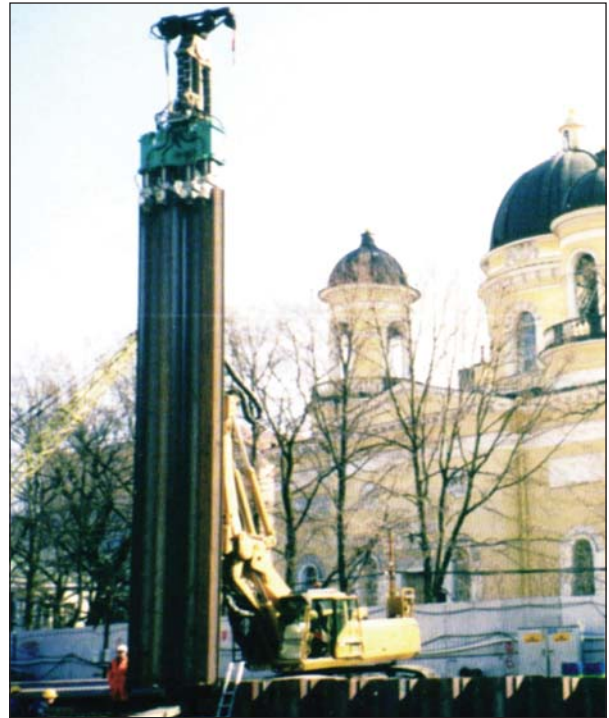
Figure 3.11 Leader mounted press
