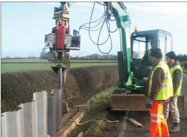
Figure 3.1 Plastic piling retaining wall installed using an EMV70 excavator mounted vibrator
