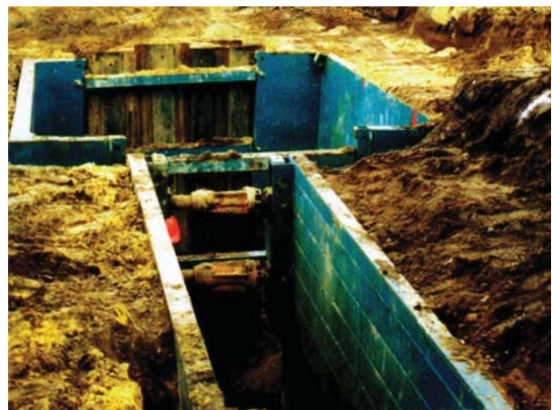
Figure 2.36 Manhole Box
