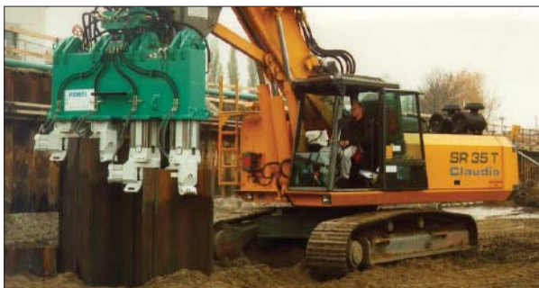
Figure 3.8 Common forms of pile presses or press systems
