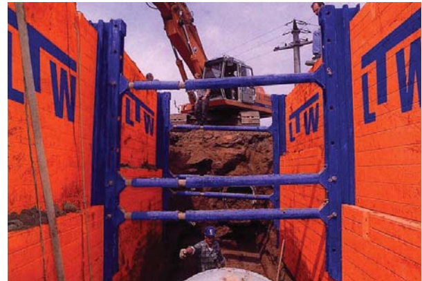
Figure 2.38 Slide rail option 3
