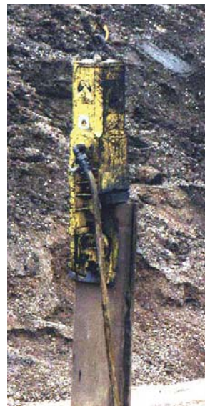
Figure 3.16 BSP 500N driving trench sheeting
