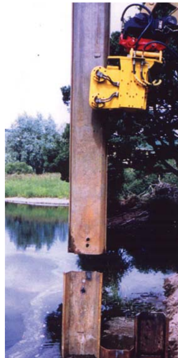
Figure 3.41 Multipiler side driving
