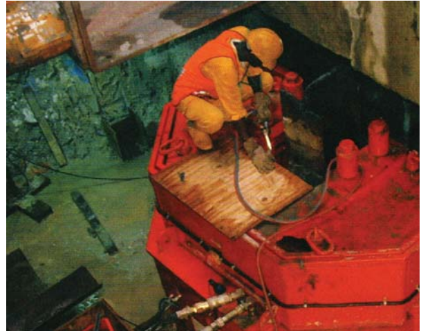
Figure 3.29 DCP Extraction Press
