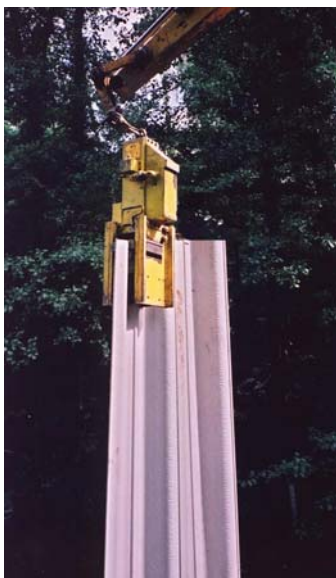
Figure 3.4 APE No.2 air hammer driving plastic piling
