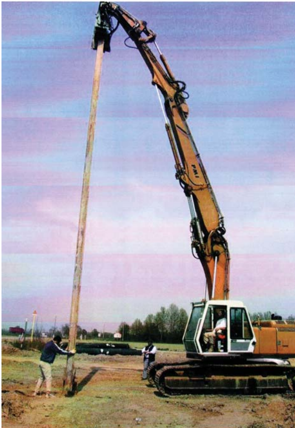
Figure 3.33 ICE SH Top Acting mounted vibrator
