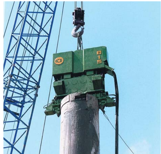
Figure 3.20 ICE 815 driving Steel Casings
