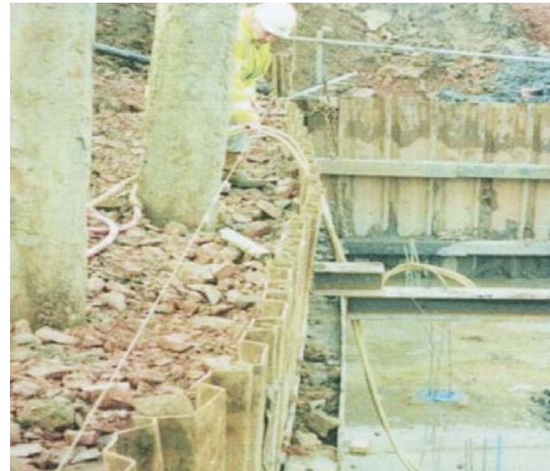
Figure 1.8 Deflection of excavation support
