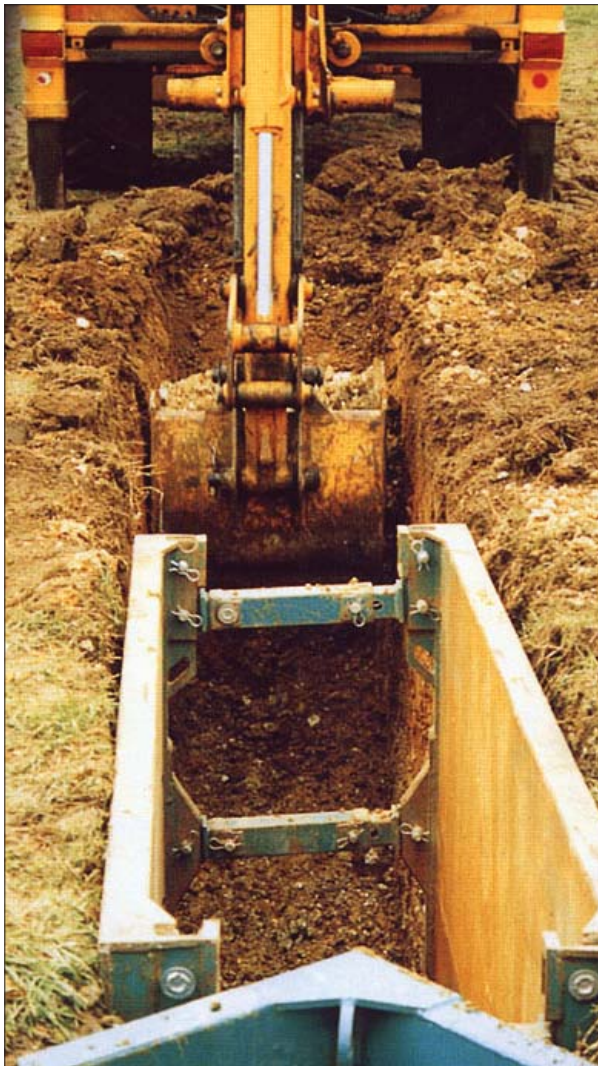
Figure 2.32 Backhoe Box Trench box
