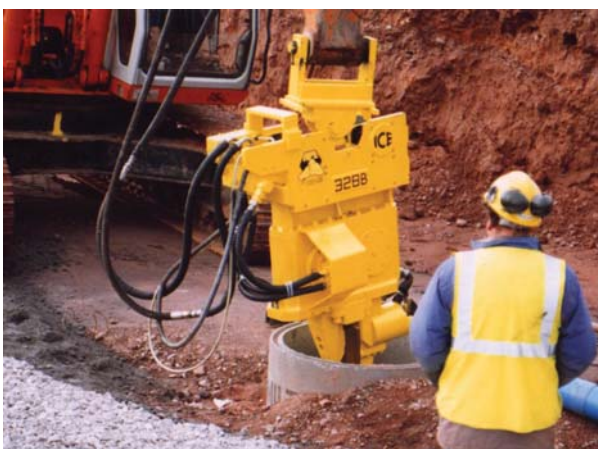
Figure 3.21 ICE 328B extracting tubes
