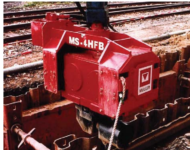
Figure 3.22 Muller MS4 extracting trench sheets
