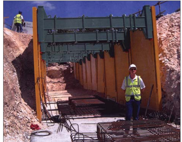
Figure 2.33 The Rolling Strut trench box - shown with high clearance positioning of rolling strut.
