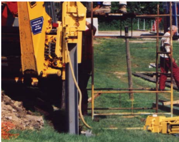
Figure 3.14 The APE No.2 driving plastic piling
