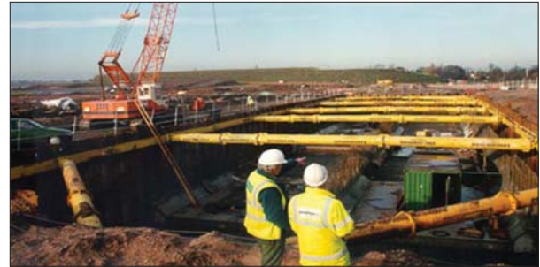
Figure 2.23 Hydraulic telescopic strut
