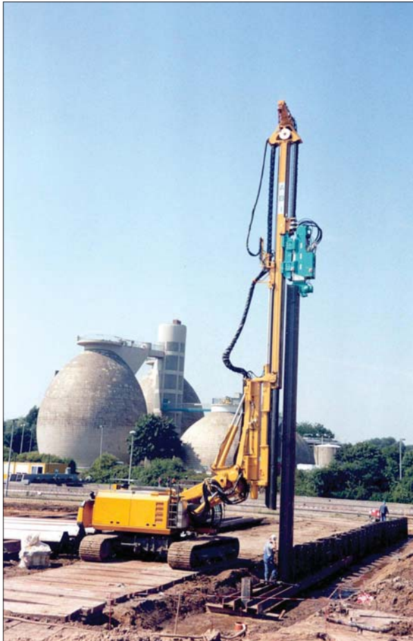
Figure 3.30 ABI Leader mounted Vibrator
