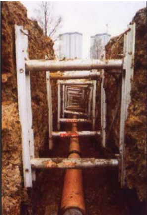
Figure 2.12 Hydraulic Vertical Shore in situ and diagrammatic representation
