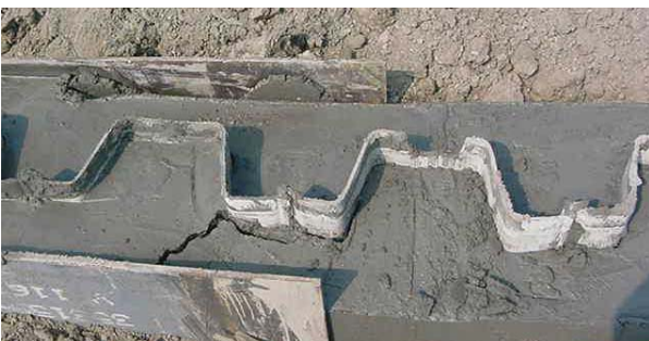
Figure 2.05 Plastic piling cut-off wall
