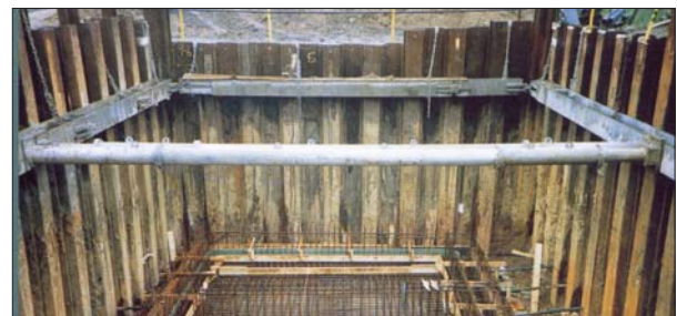
Figure 2.25 Hydraulic telescopic strut
