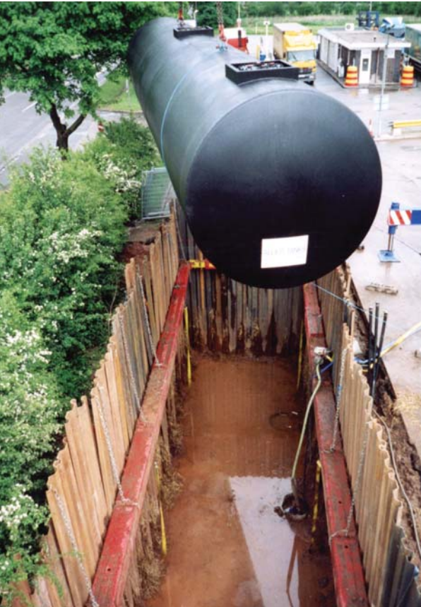
Figure 2.19 Hydraulic Bracing Frame - Double acting brace.
