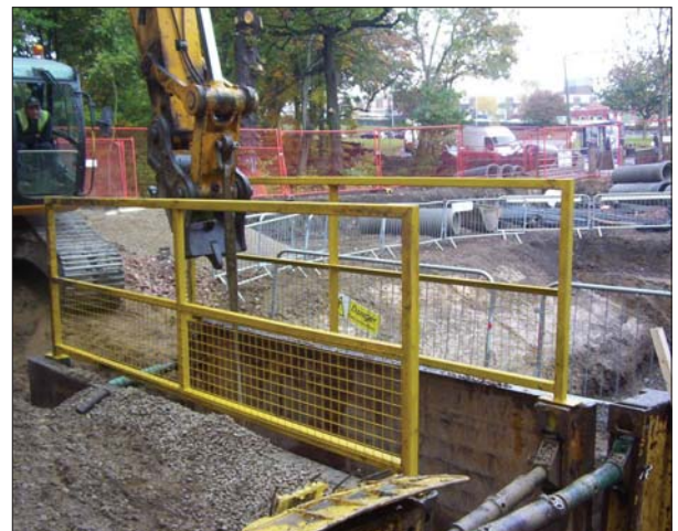
Figure 2.33 Proprietary edge protection to a trench box.
