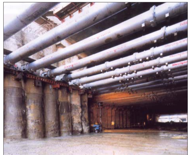
Figure 2.26 Hydraulic telescopic strut used with in situ concrete piling .
