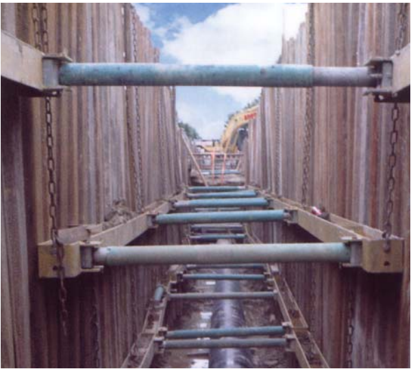
Figure 2.14 Hydraulic waler frame in situ
