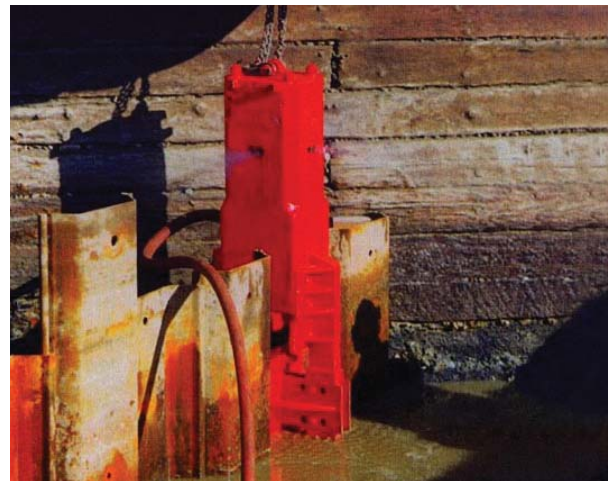
Figure 3.2 BSP 500N driving steel sheet piling
