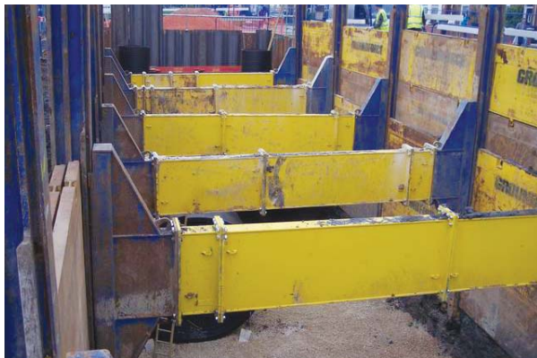
Figure 2.37 Slide rail Option 2 Rolling Strut
