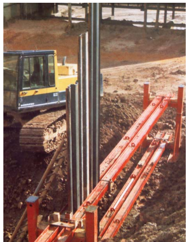
Figure 2.10 Piling Trestle used for Trench Sheetting
