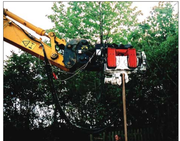
Figure 3.32 EMV300 excavator mounted via a Powertilt
