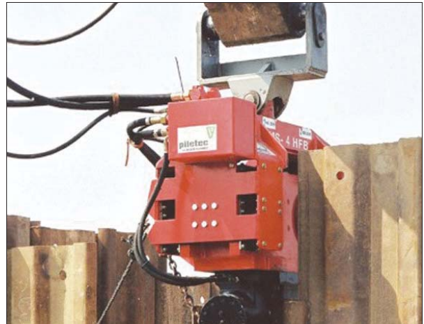
Figure 3.35 EMV 300 driving trench sheets
