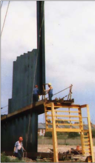
Figure 2.11a Piling Trestle using a Leader rig
