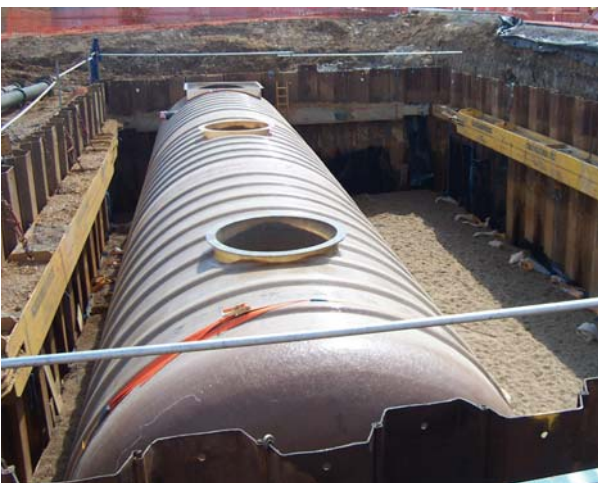
Figure 1.3 A 22m long prefabricated tank installed in a braced excavation
