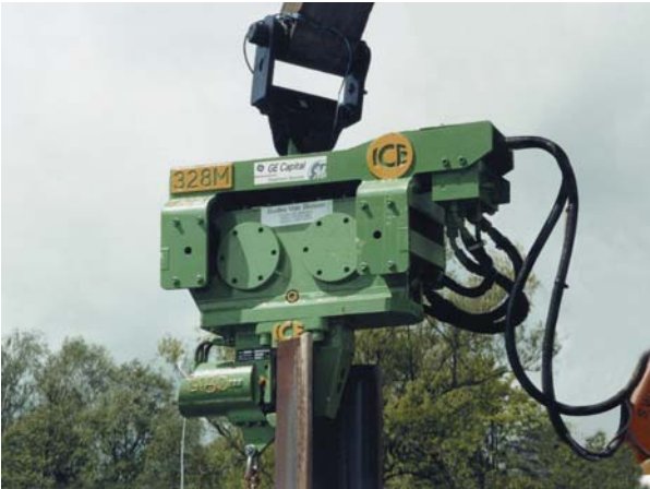
Figure 3.6 ICE 328M excavator mounted vibrator driving steel sheet piling
