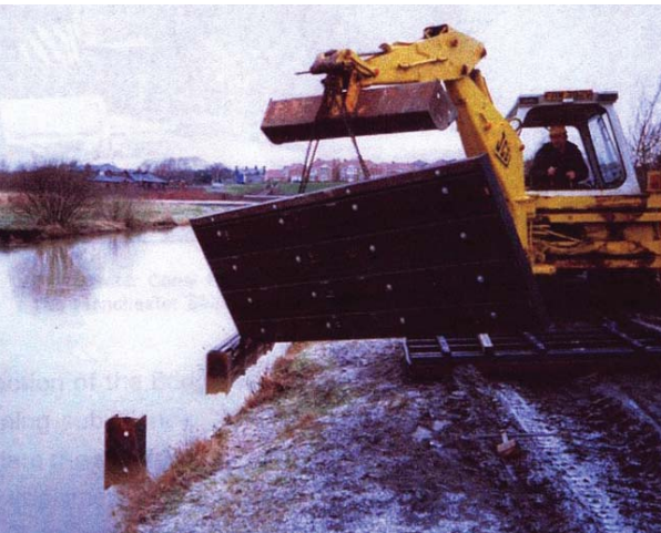
Figure 2.41 King Post using reinforced PVC panels
