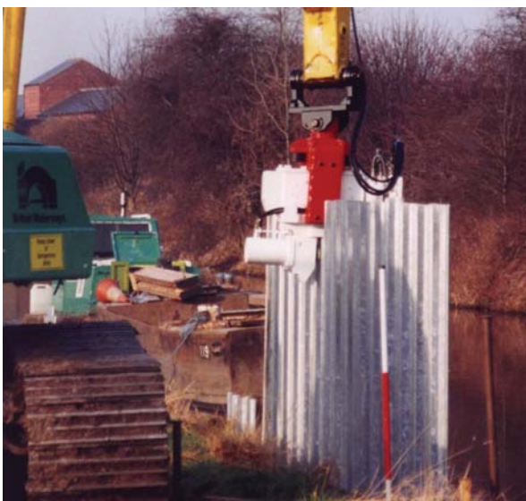
Figure 3.7 EMV70 driving interlocking trench sheeting
