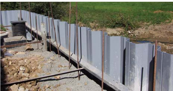
Figure 2.04 Plastic piling retaining structures
