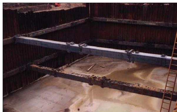
Figure 2.22 Hydraulic telescopic strut
