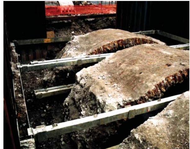
Figure 2.06 300kN Bracing Struts used in singles and pairs
