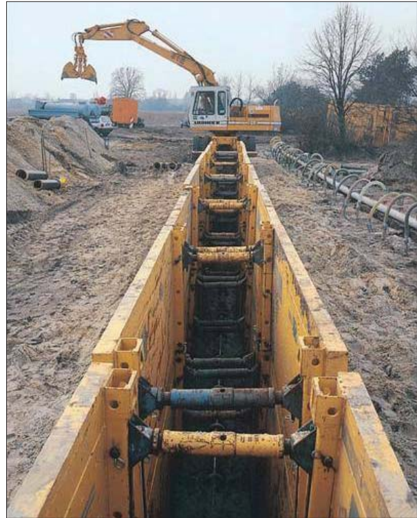
Figure 2.28 Trench box, trench lining
