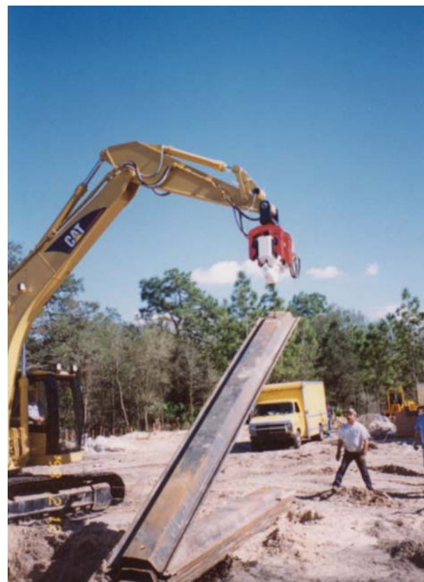
Figure 3.3 EMV300 excavator mounted vibrator pitching trench sheeting
