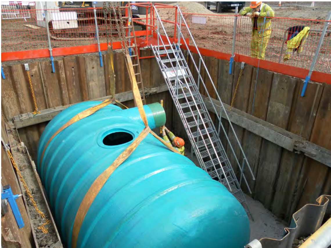
Figure 1 - Safe Access into an Excavation
