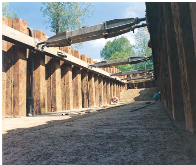
Figure 7 - Proprietary Bracing Strut
