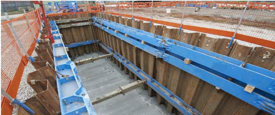
Figure 6 - Proprietary Shaft Bracing System
