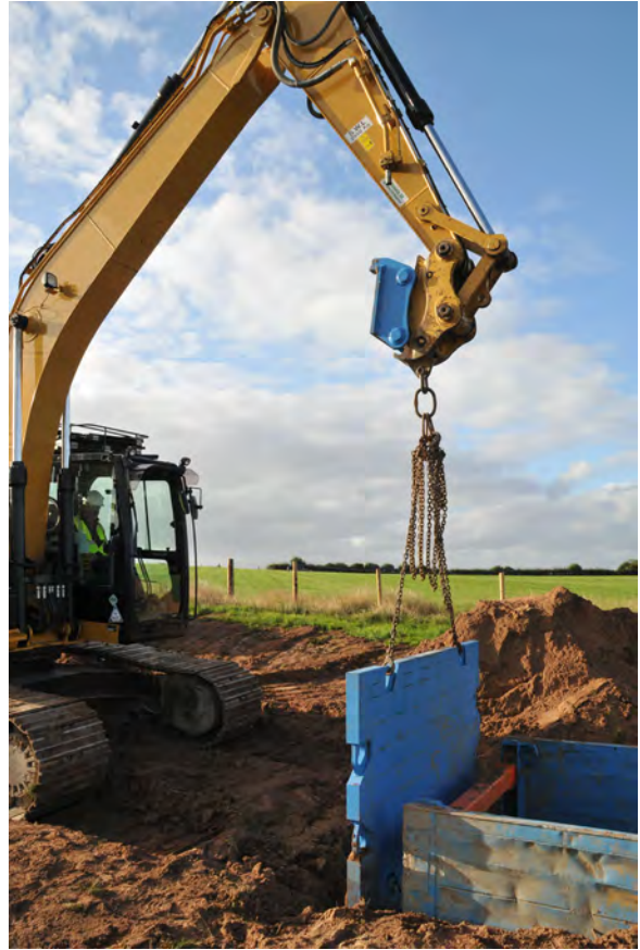
Figure 3 - End Panel Installation
