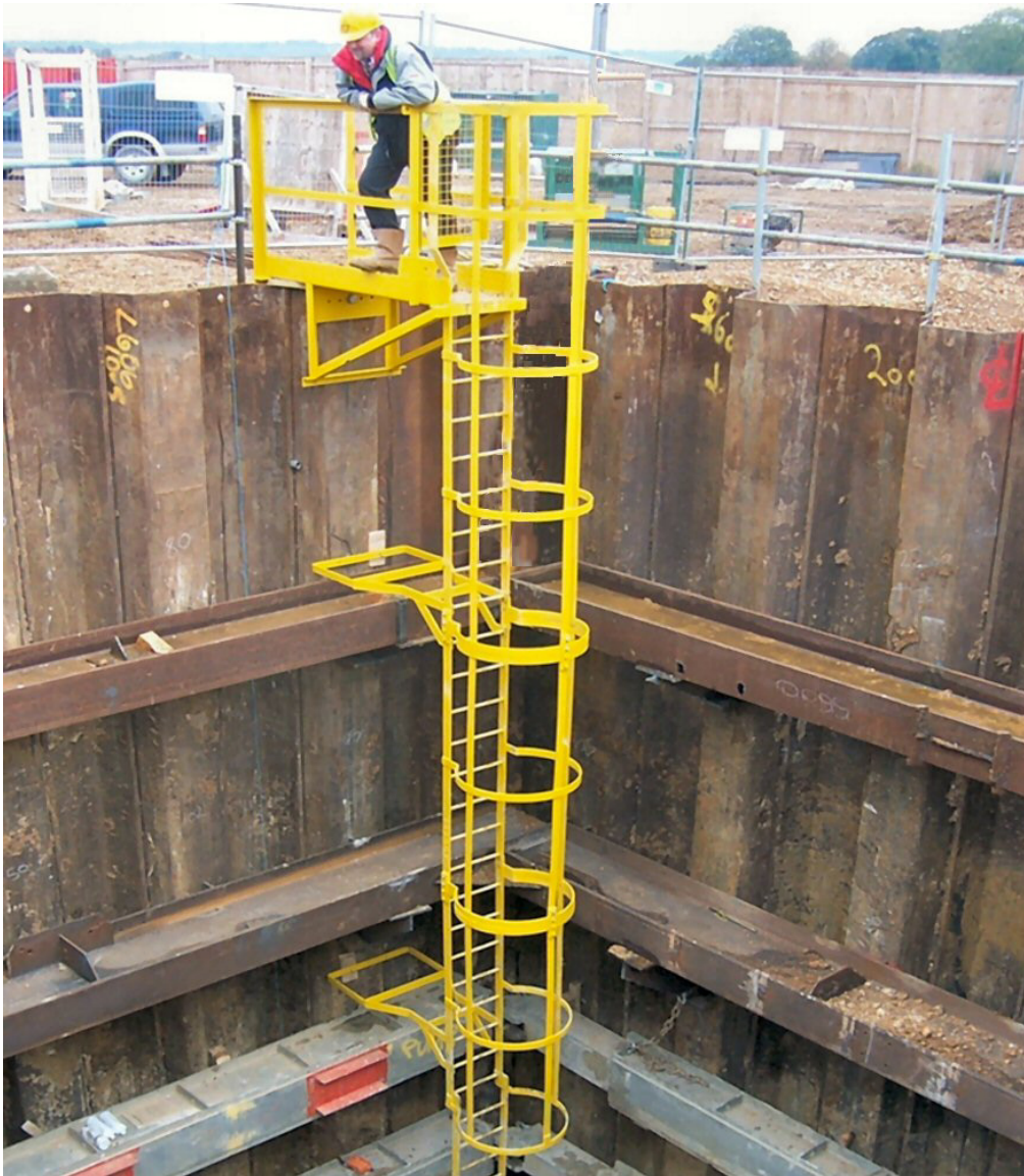
Figure 3 - Example of a safety ladder in a deep cofferdam
