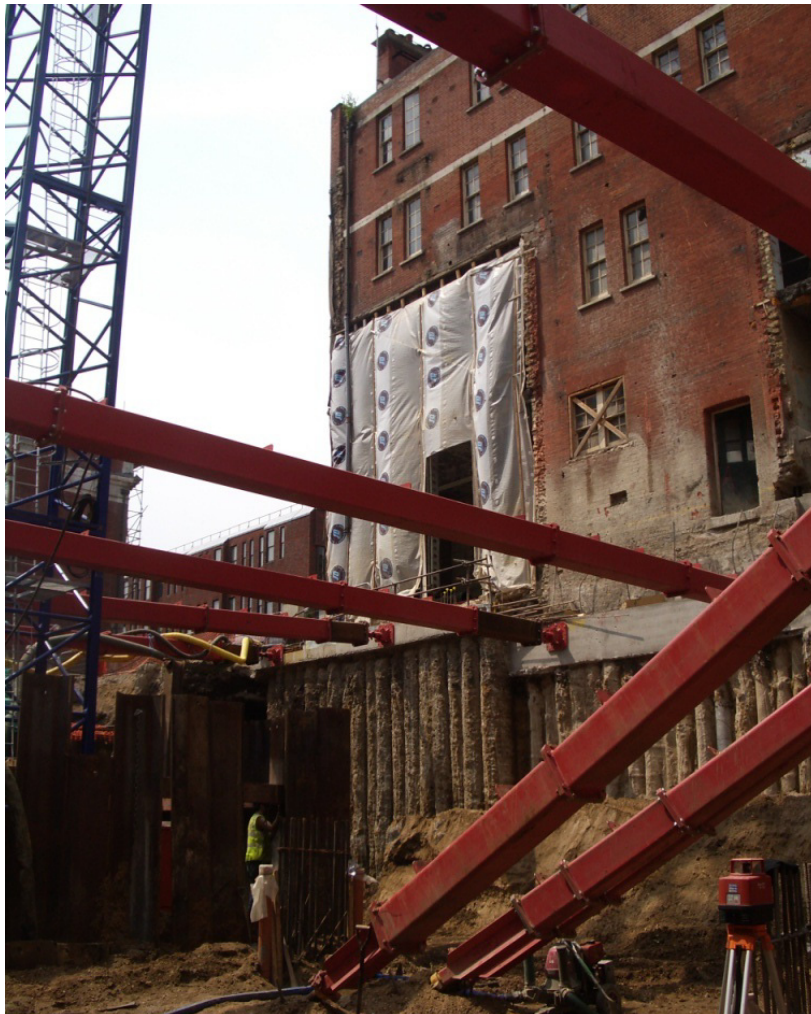
Figure 5 - Risk Level 3 Excavation Large, complex and high risk to life and property
