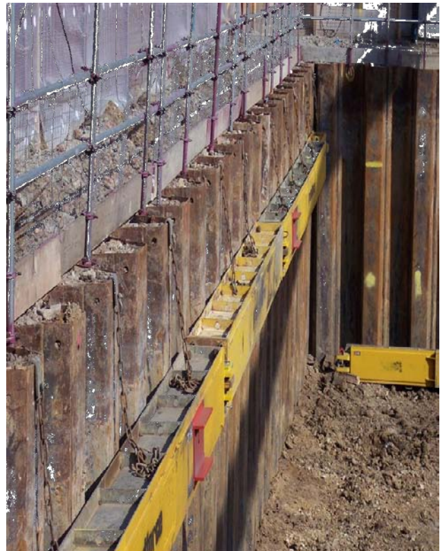
Poor Installation – Angle Greater than 30°
