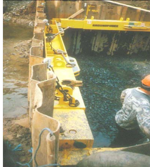
Poor Installation – Angle Greater than 30°
