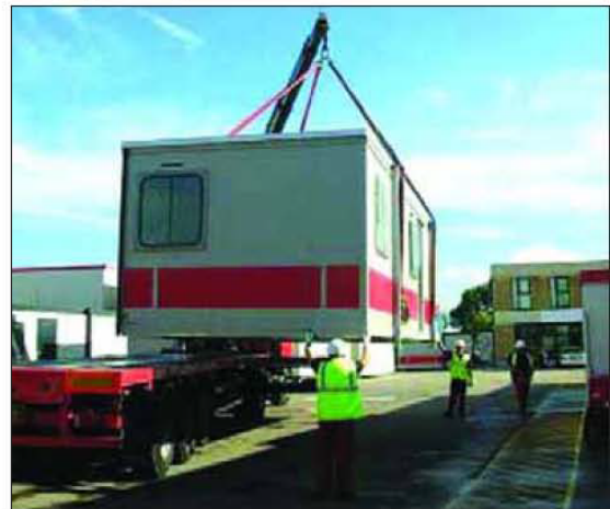
Figure 2 A successful lift with slings in place
