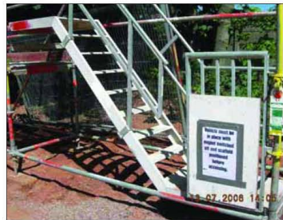
Figure 3 Safe stair access onto the scaffolding system
