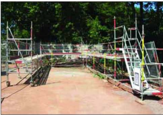
Figure 2 System scaffold unloading gantry
