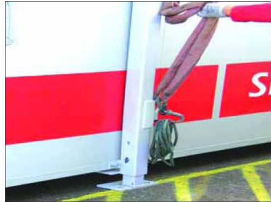
Figure 5 Lifting jackleg cabins from the base, removing the need for people to access the roof of the cabin or vehicle.
