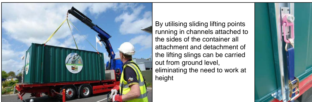
Example of Eliminating the Need for Work at Height
